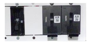
The breakers at the bottom of the power distribution panel (PDP) are for the battery bank. In this photo, the one on the left is for the charge controller, and the two on the right are for the inverters. In the event of battery failure, these should all be turned off.
