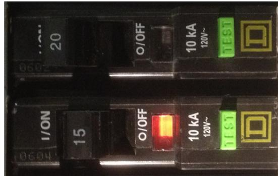
The image above shows two breakers. The top one is ON and normal, the bottom one is tripped. The handle will be more centered and orange can be seen through the window to indicate that it had tripped. To reset a tripped breaker, correct the overload situation, and then switch it all the way to the OFF position, and then back ON.
