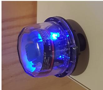
Each suppression device has two blue LEDs inside. When the sun is shining, these LEDs will both be lit. If at any time you notice one or both LEDs not lit and the sun is shining, contact mtvSolar for inspection.
