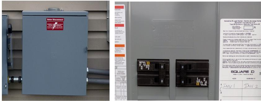
The combiner will contain circuit breakers, one for each inverter. During normal system operation, all breakers should be ON.
